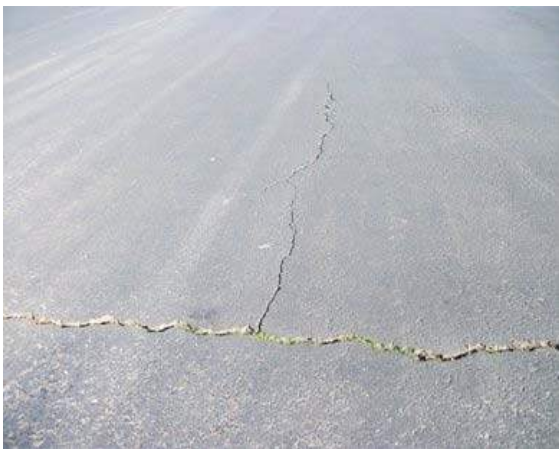
Unsealed Cracks
