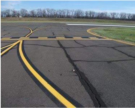
Widening of Sealed Cracks
