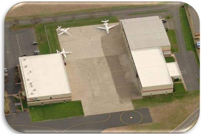
Conventional Hangar at Bradley
