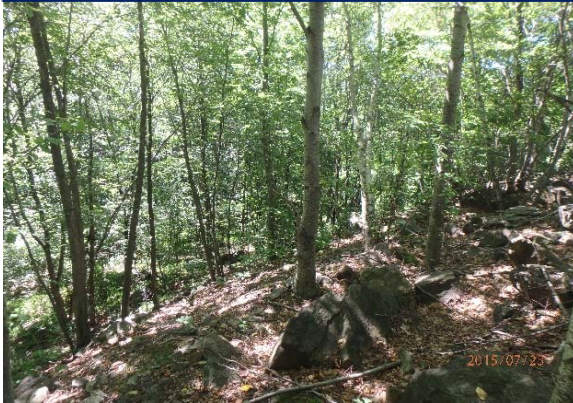
Rocky Fill Slope on Western Edge of Parcel 9
