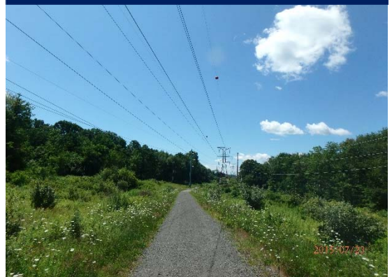
Power line right-of-way at Parcel 12
