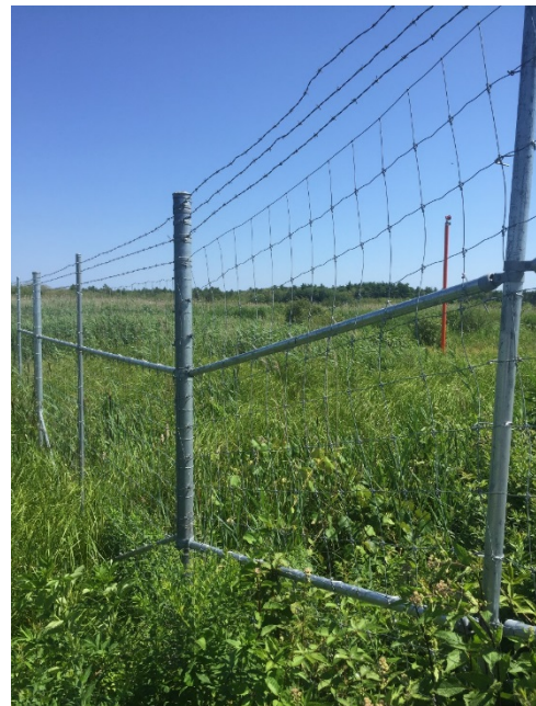
Woven wire fence at New Bedford Airport, MA (fence shown with barbed wire along the top, no barbed wire is proposed for GON fence)
