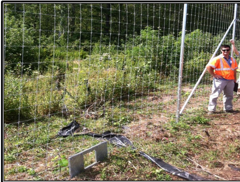
Photograph No.: 12 Wildlife deterrent fence at New Bedford airport with turtle inclusion device
