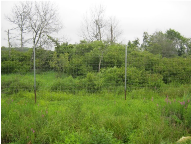
Woven wire fence installed at Norwood Memorial Airport, MA (fence shown is 10-feet high, proposed fence at GON would be 8-feet high)
